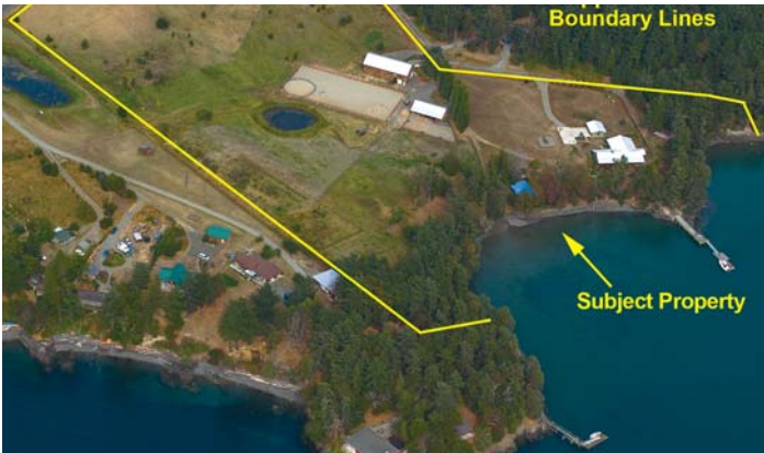
EXQUISITE WATERFRONT ESTATE. Four waterfront parcels totaling 18± acres with over 1000' of shoreline; a 3555± sq ft timber peg home, two waterfront cabins, private dock, 5600± sq ft shop/barn, horse barn and riding arena. #28021162 $3,950,000 www.SamBuck.com and Nancy Young
